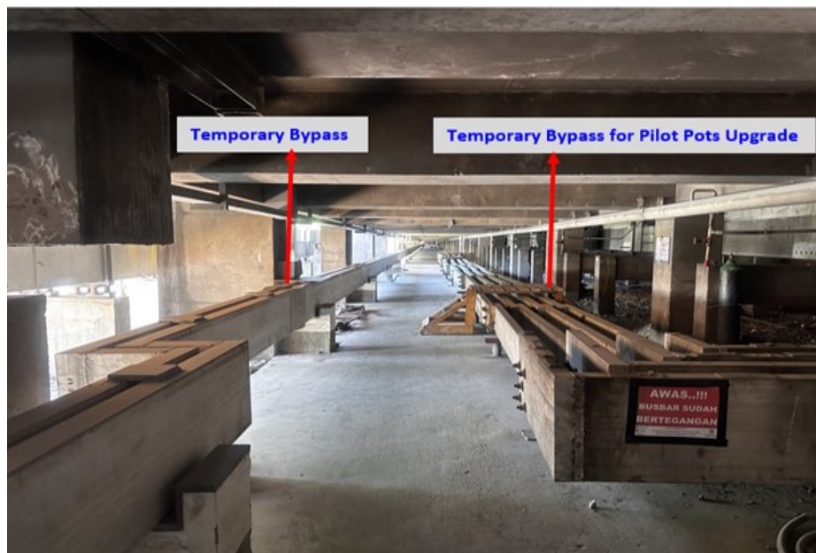
Figure 3. Temporary bypass for the construction of the pilot cells.
