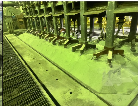
Figure 8. Cell sealed with crushed bath and ready for hooding and energization.
